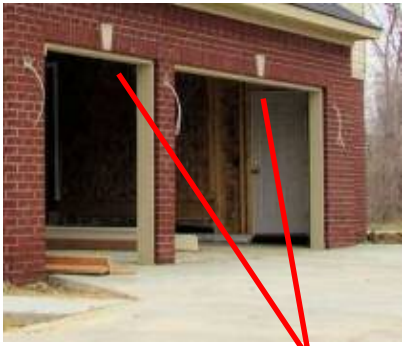
10" Keystones over side entry garage doors
