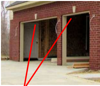
10" Keystones over side entry garage doors
