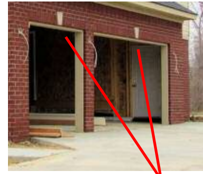
10" Keystones over side entry garage doors
